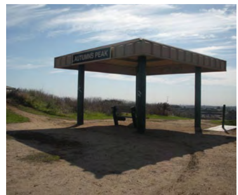
Shade structure and interpretive view point at the top of the Western Ridgeline.
