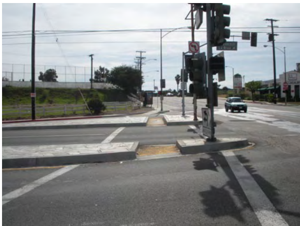
The vehicle dominated Five Points intersection has pedestrian activated signals and some existing curb ramps. Curb cuts are needed at the northeast corner of Stocker and La Brea. The crossings would need to be improved to meet ADA standards.
