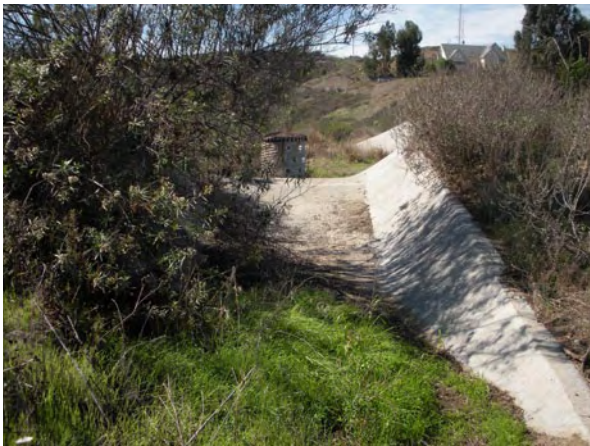
Concrete drainage ditch on the BHRCA property
