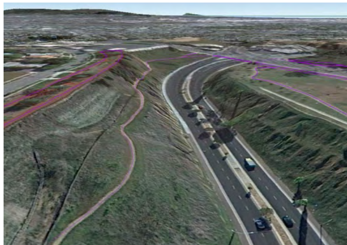
Looking west along Stocker Street, Ruben Ingold Park is located at the top of the slope, Stocker Corridor Trail runs parallel to Ingold park down slope, and Norman O. Houston park is located across the valley of Stocker Street.
