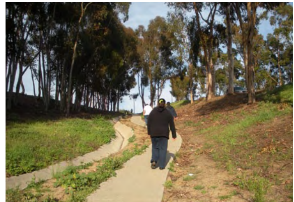
Concrete sidewalk with concrete drainage v-ditch leads from the lower picnic area up to Janice's Green Valley.
