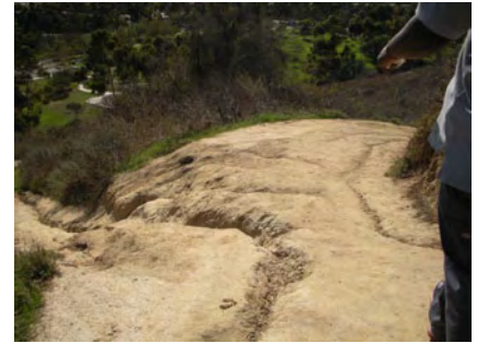
Areas with steep running slopes have lead to deep runnels from water eroding the trail surface.
