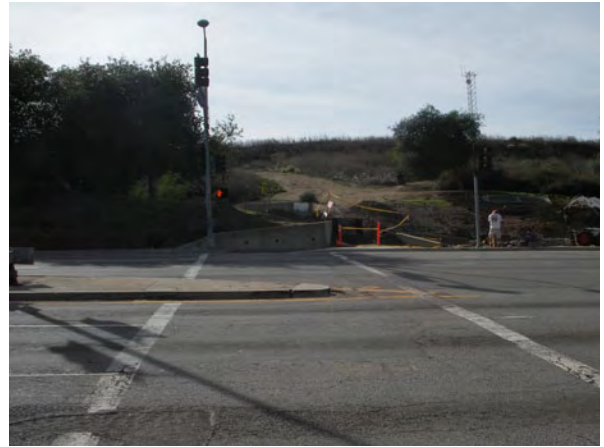
The Eastern Gateway provides a formalized entrance to KHSRA at Don Lorenzo Drive, however it is not ADA accessible.
