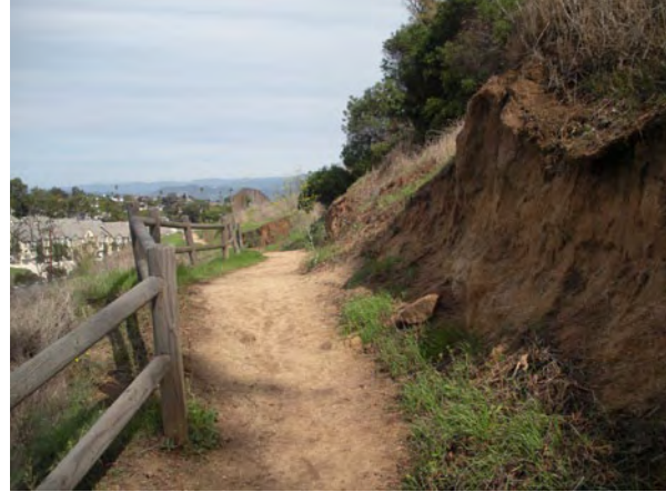
Example of erosion of the top bank where the trail has been cut into a slope. A split rail fence is a barrier to the steep slope below.
